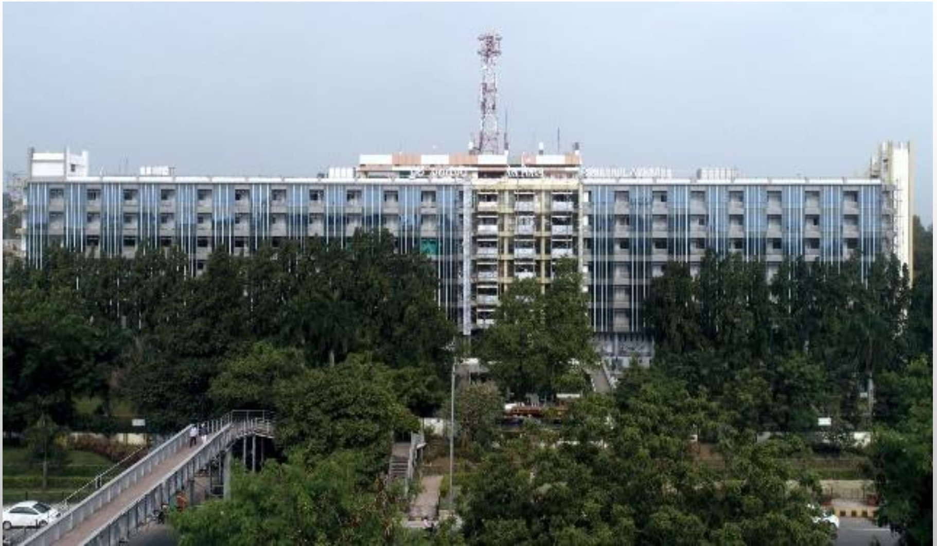
Rail Nilayam, General Manager's Office, South Central Railway, Secunderabad
